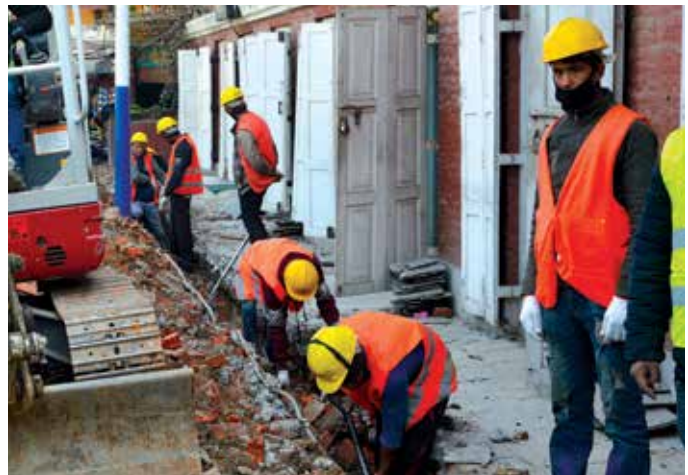
■ Workers laying Melamchi Project pipeline at Durbarmarg, Kathmandu.
