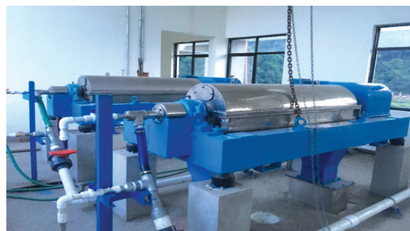
Centrifuge installed at Guheshwori WWTP
