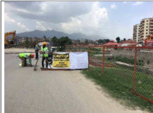
Laborer erecting safety barrier at -TP-02
