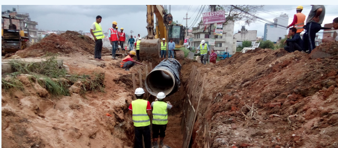
Pipelines being extended at Koteswar-Balkumari road section
