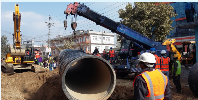
Pipeline being laid at the Mahankalchaur-Arubari road section
